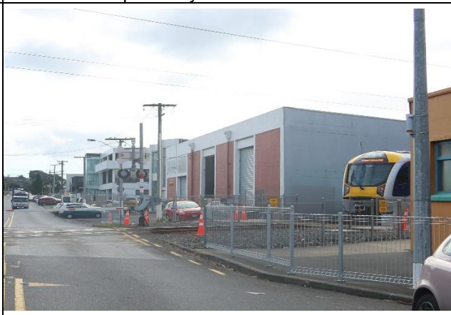
View of signalling when crossing is activated on the wrong side of the road (half-arm barrier has very low visibility and flashing lights are not observable)
