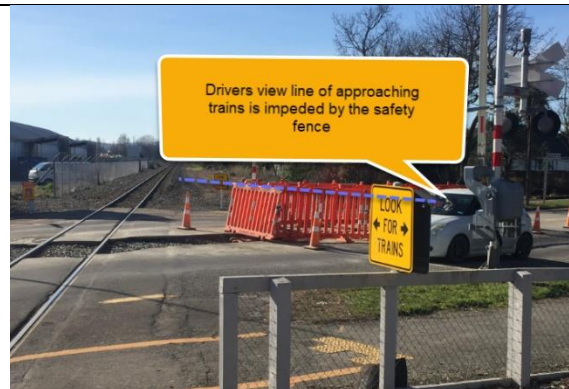
Example of driver view lines where fencing is used in proximity to the rail corridor
